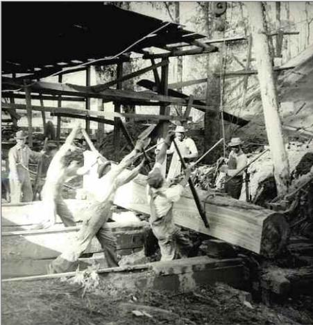
These three photos are all from Beal Lumber Company sawmills. This one was taken in 1950. The workers are using cant hooks at a steam-powered (“Push-Hard”) mill on Wadmacon Island, Santee Delta, in Georgetown County, S.C.
