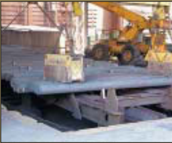
...where they are readied for reheating.
