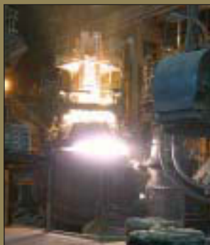
...which are then loaded with scrap steel in precise grades and turned into molten metal, whereupon the mixture is electromagnetically stirred and chemically adjusted to create the exact recipe for making a variety of products, including rail.
