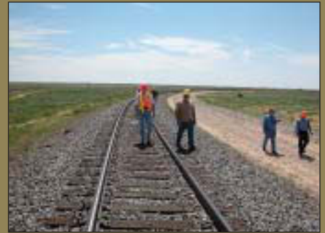
A final track walk on the FAST track gives the attendees opportunity to see all the configurations of tie species and fasteners.
