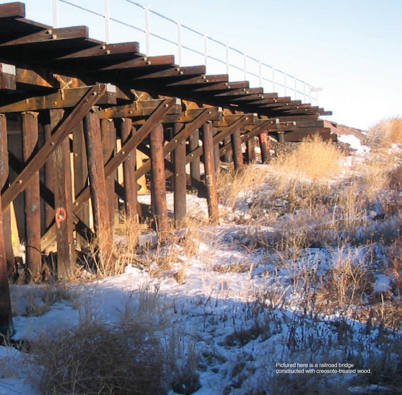
Pictured here is a railroad bridge constructed with creosote-treated wood.
