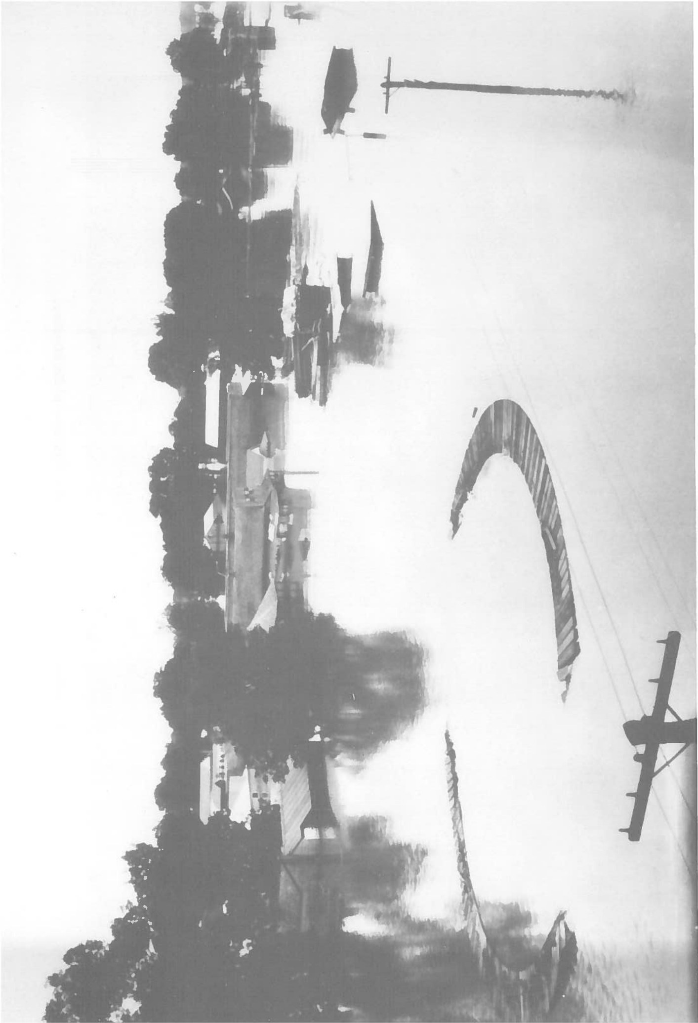
A floating wood tie turntable - Holly Bluff, Mississippi - 1927. Courtesy of Ed Brindley.
