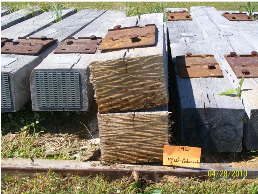
Figure 59 - Tie #190 (Cedarcide/white oak) with decayed areas marked.
