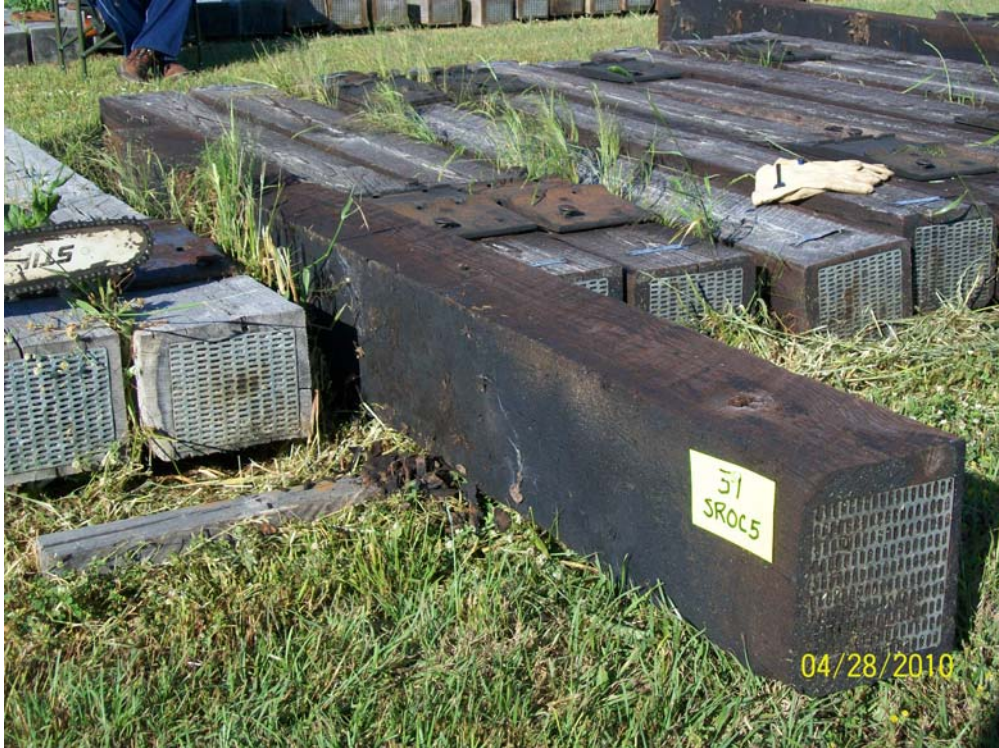
Figure 7 – Tie #31 (Boatright/red oak/creosote 5pcf).
