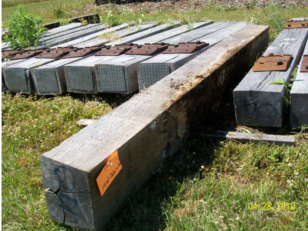
Figure 58 - Tie #190 (Cedarcide/white oak) with decayed areas marked.
