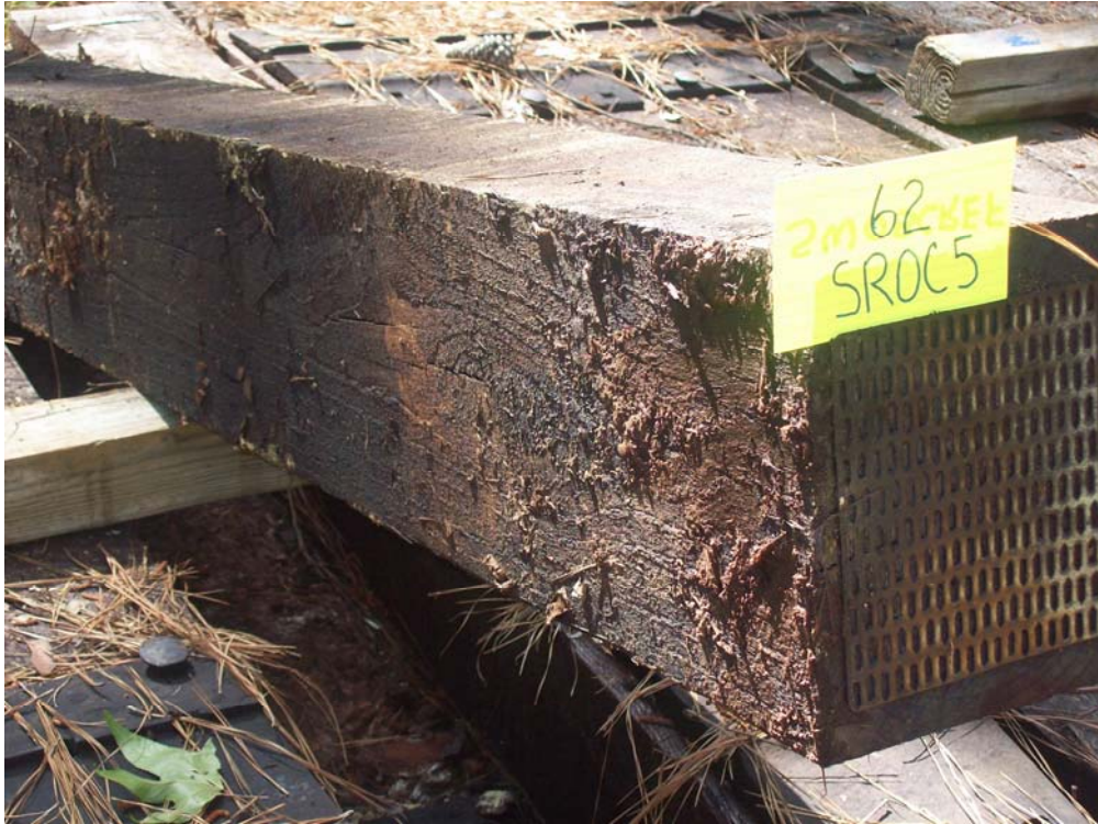
Figure 45 Tie #62 (Boatright/red oak/creosote 5pcf).
