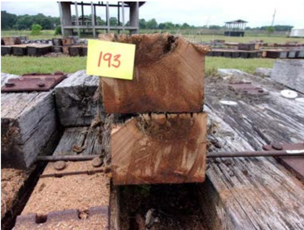
A106 - Tie #193 (Cedarcide/white oak) internal decay.
