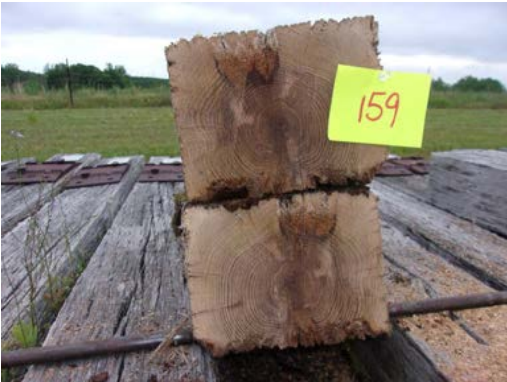
A102 - Tie #159 (Nisus/white oak/boron) with decay around checks.
