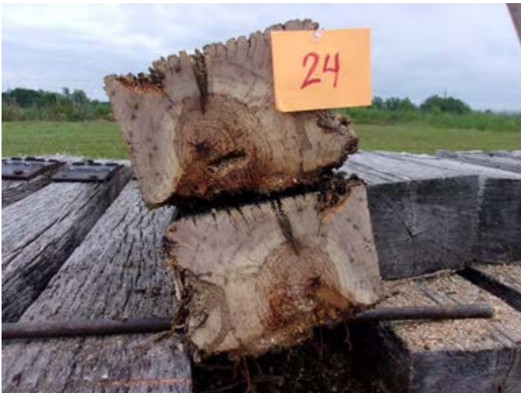
A70 – Tie #24 (Envirosafe/white oak) with extensive decay.
