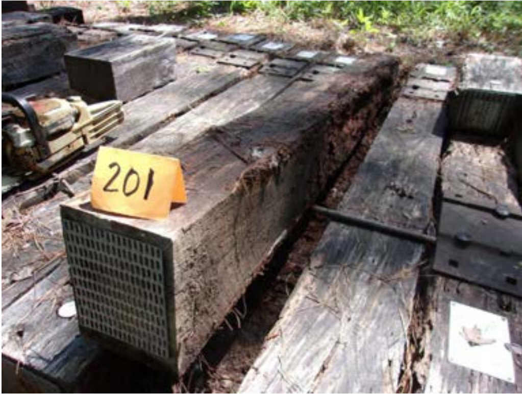
A39 - Tie #201 (Nisus/red oak/borate) decay & trace termite attack on bottom.
