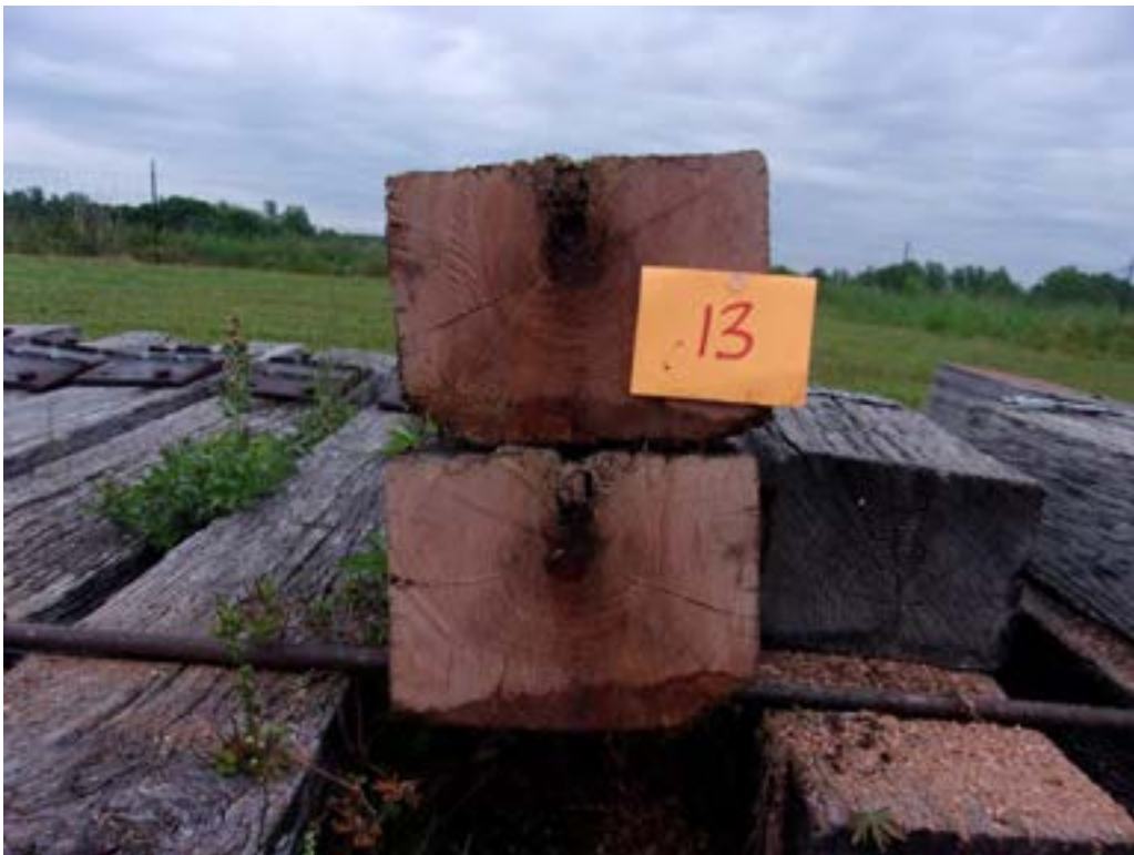
A68 – Tie #13 (Envirosafe/red oak) with decay.
