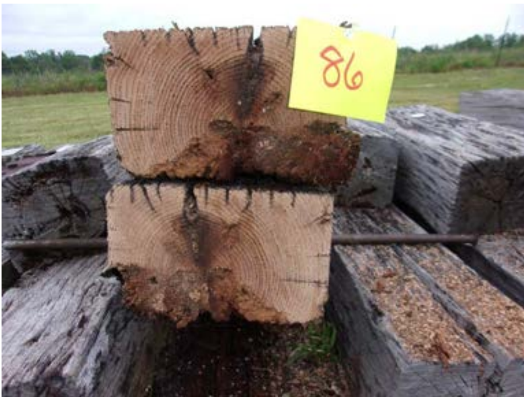
A82 - Tie #86 (Lonza/red oak) heavy decay evident in cross-section.
