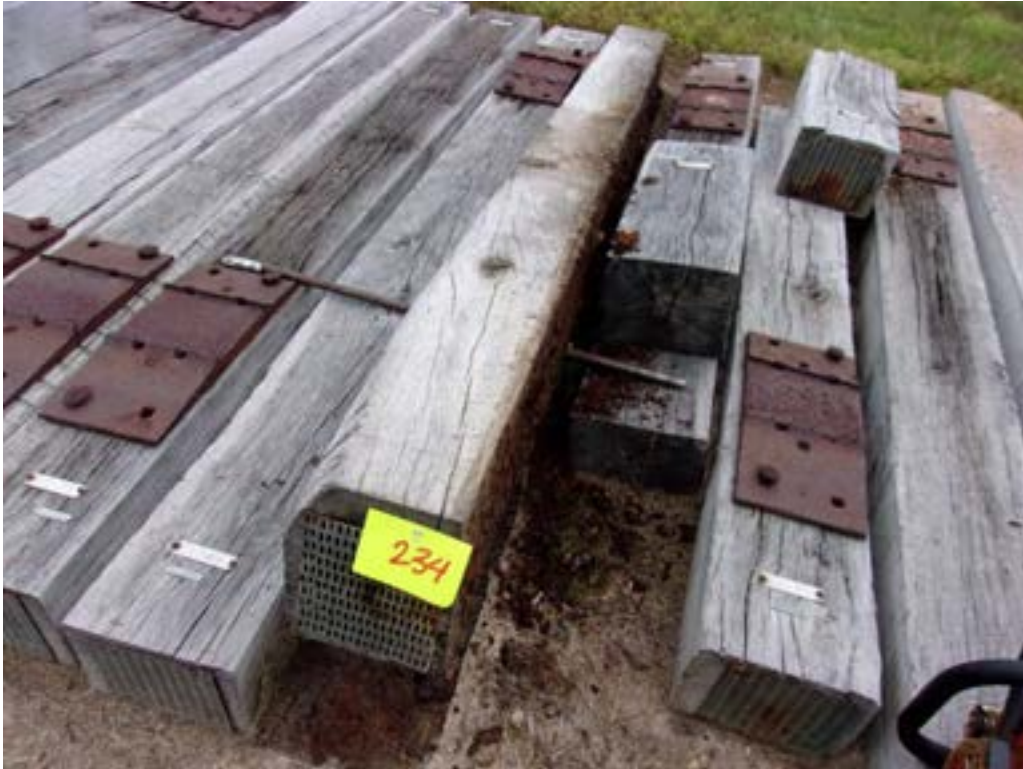
A113 - Tie #234 (Merichem/white oak/CuNap) with decay & Formosan termites.
