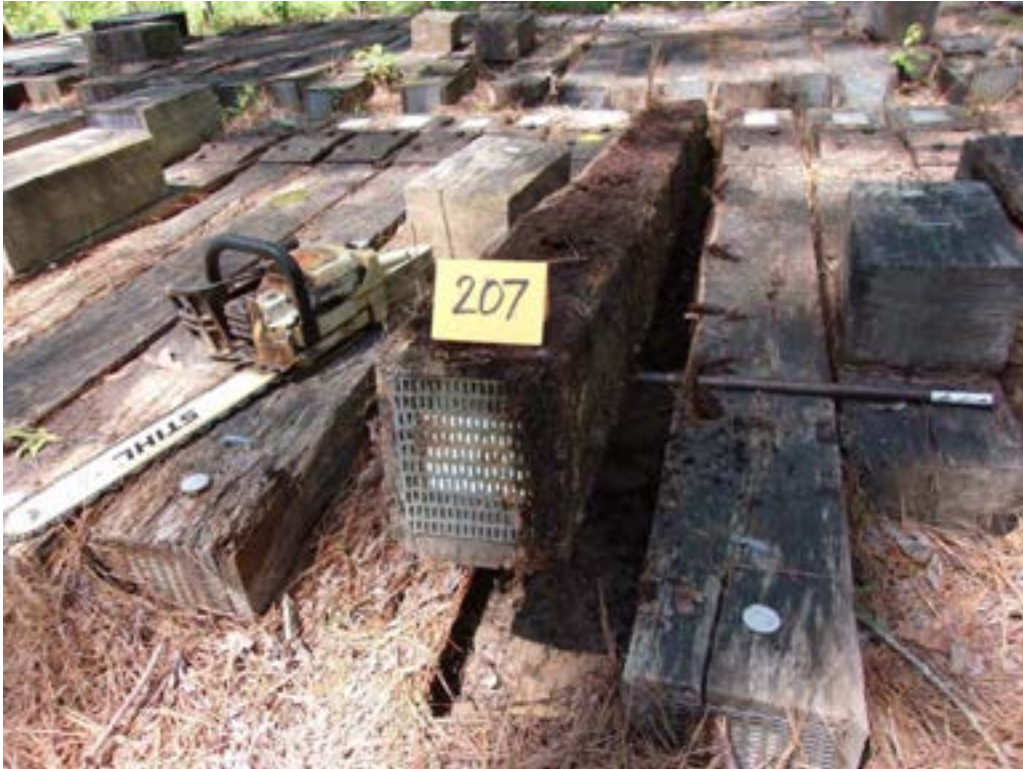
A41 - Tie #207 (Nisus/white oak/borate) with light decay on bottom.
