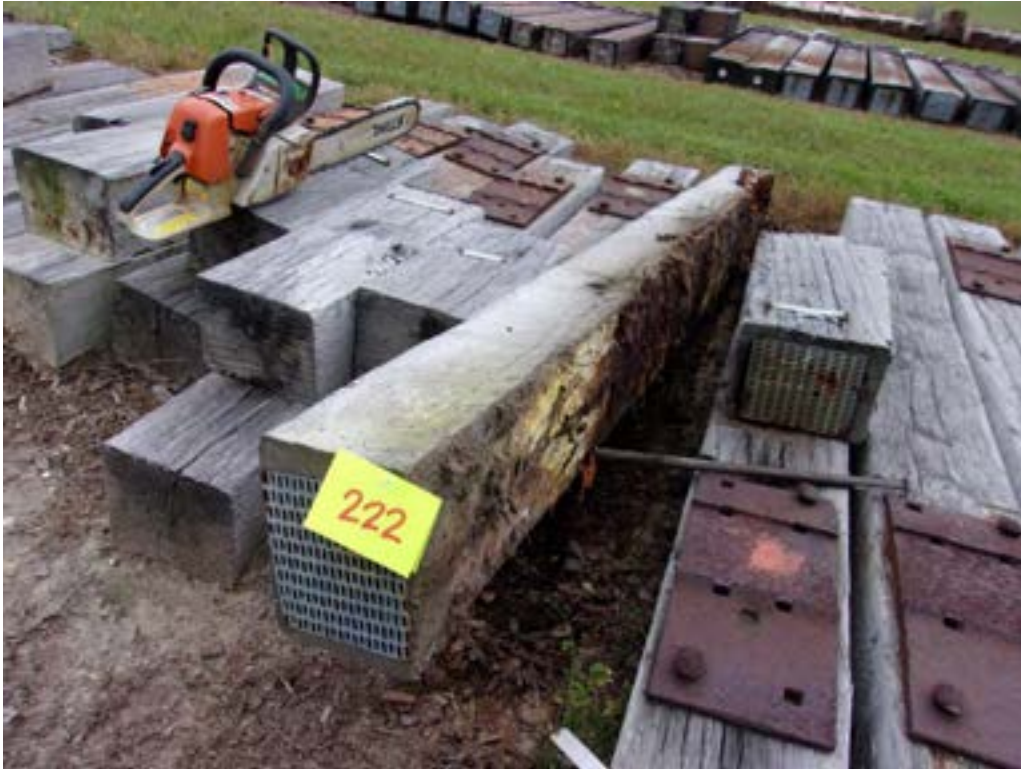
A111 - Tie #222 (Merichem/red oak/CuNap) with decay & Formosan termites.
