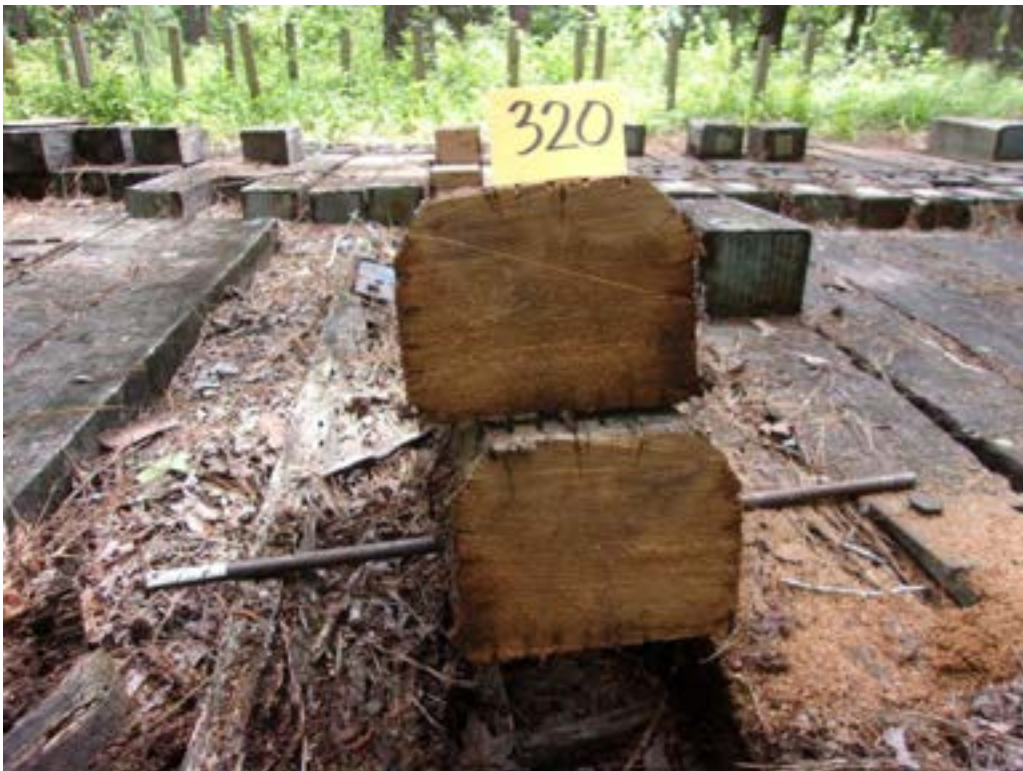
A46 - Tie #320 (untreated/white oak) with decay.
