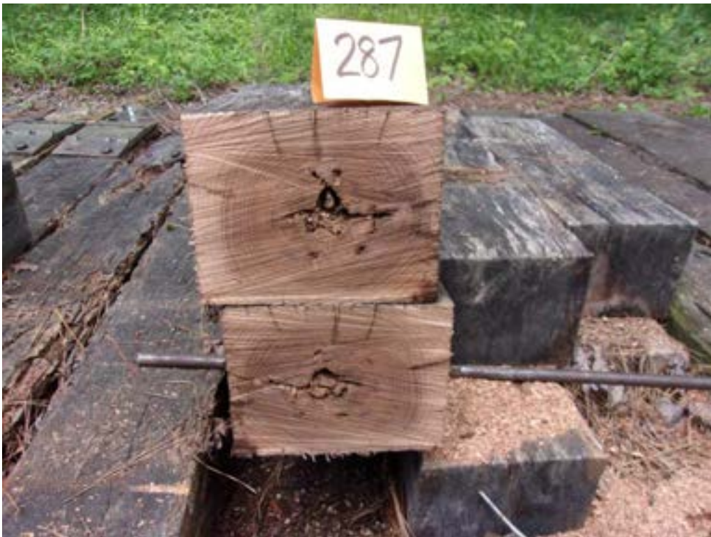
A62 - Tie #287 (Envirosafe/red oak) with decay on bottom & internal.
