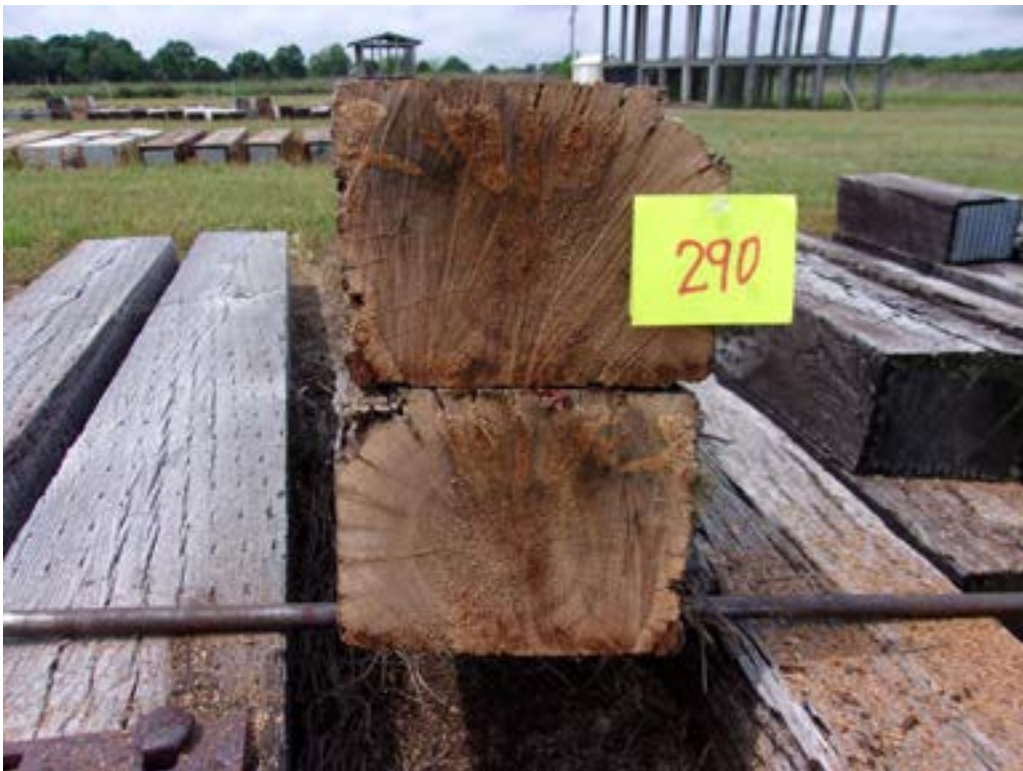
A96 - Tie #290 (untreated/white oak) with decay.
