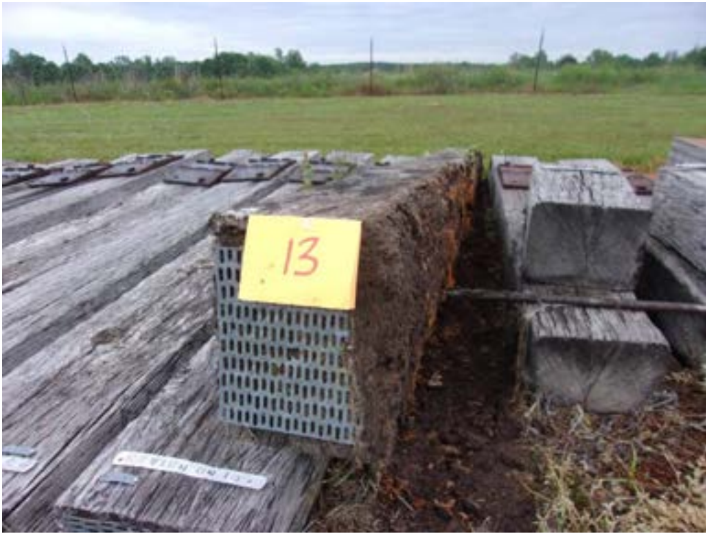
A67 – Tie #13 (Envirosafe/red oak) with decay.
