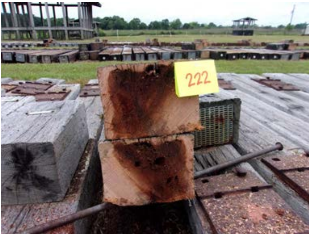
A112 - Tie #222 (Merichem/red oak/CuNap) with internal decay.
