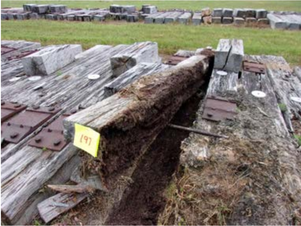
A107 - Tie #197 (Cedarcide/red oak) with extensive decay on bottom and side.
