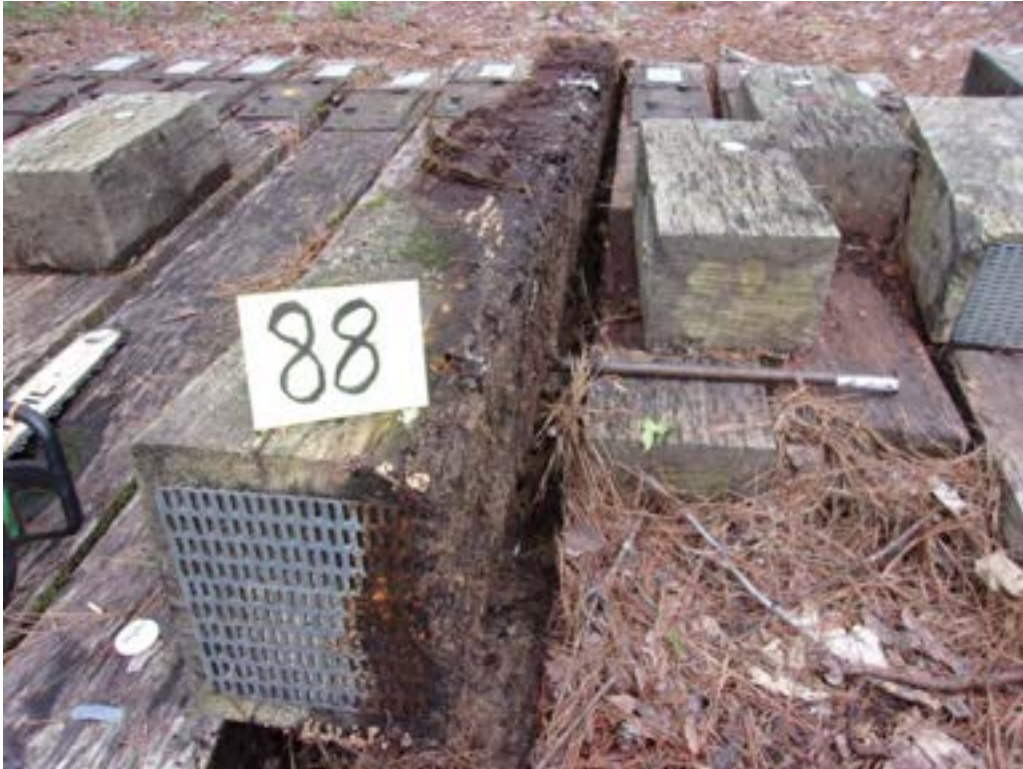
A17 - Tie #88 (Lonza/white oak) decay on bottom.
