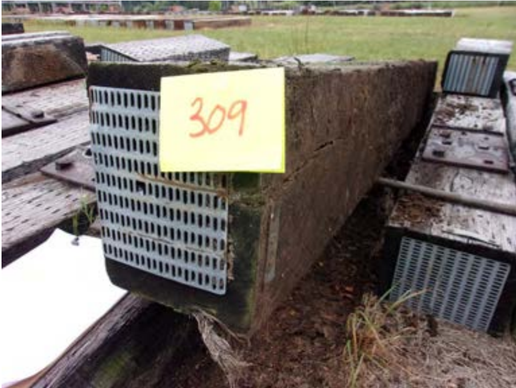
A125 - Tie #309 (Koppers/white oak/creosote petroleum solution) with trace Formosan termite damage.
