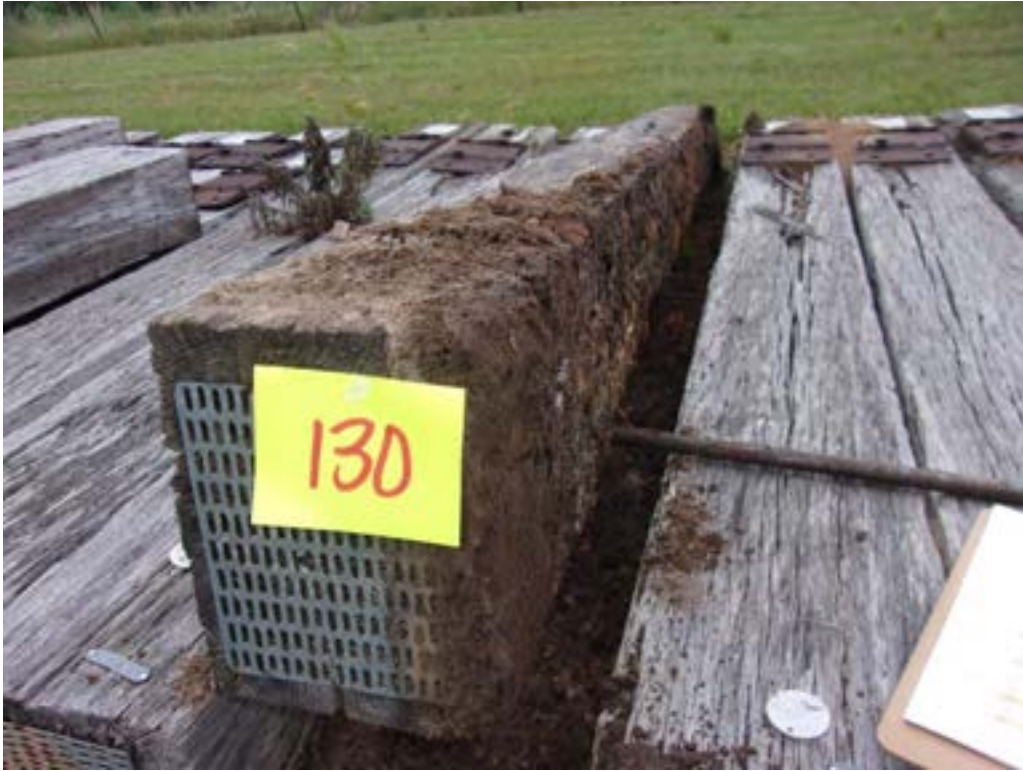
A89 – Tie #130 (Nisus/red oak/borate) with decay on bottom.
