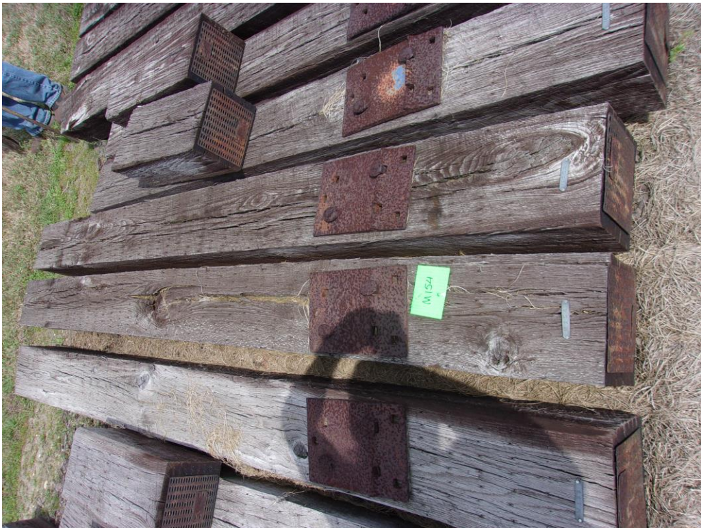
Figure 7 – Tie 154 with large check holding moisture.
