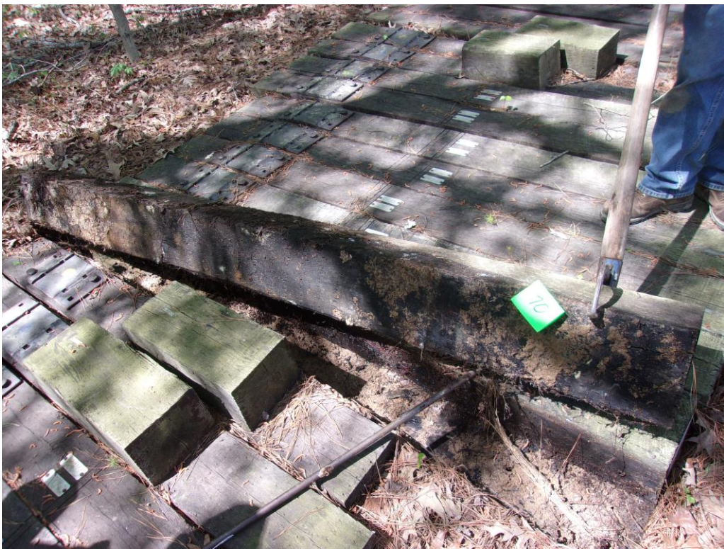
Figure 3 - Tie 70 showing no signs of decay or termite damage.
