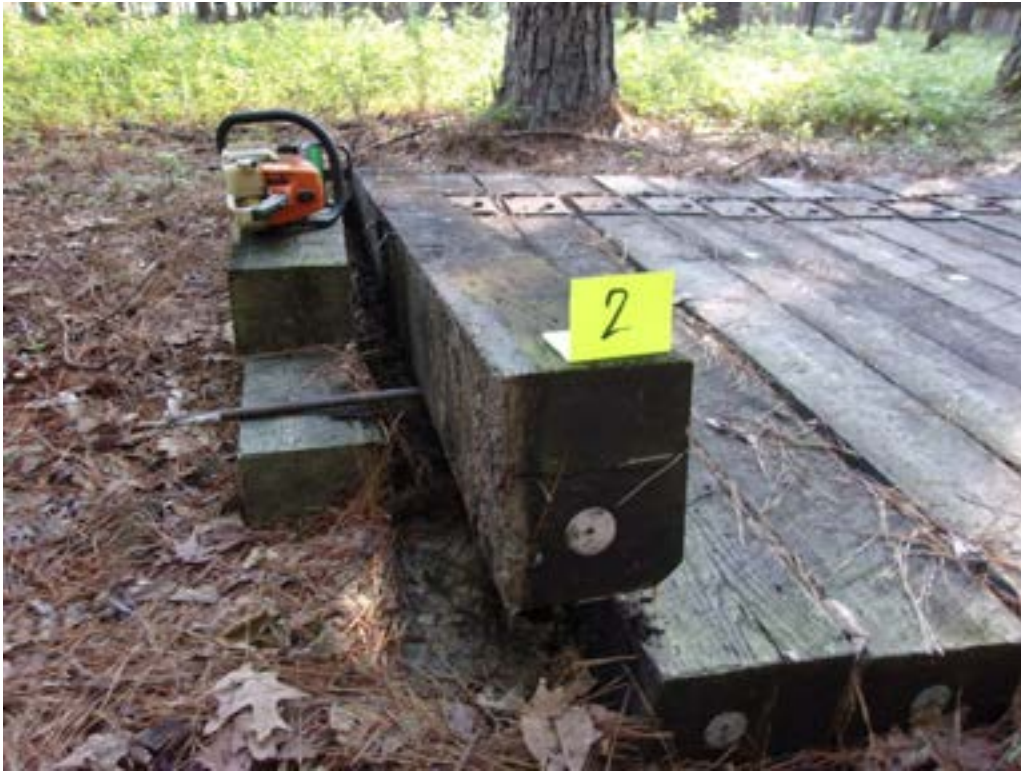
Figure 1 - Tie #2 white oak/borate/creosote 6# (Koppers).
