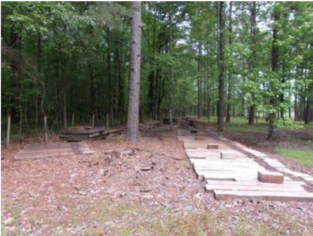
Figure A - Site 1 (MSU Dorman Lake Test Site) at the time of inspection.
