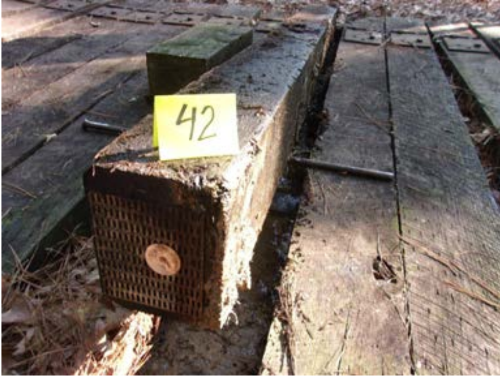
Figure 9 - Tie #42 white oak/borate/creosote 7lbs (Koppers).
