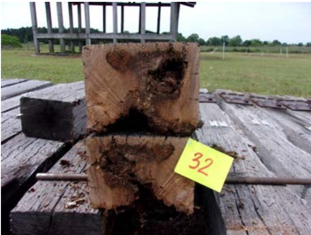
Figure 60 - Tie #32 untreated white oak with extensive decay.
