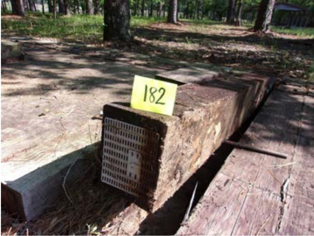
Figure 39 – Tie #182 Douglas fir/P2 creosote (Lonza).
