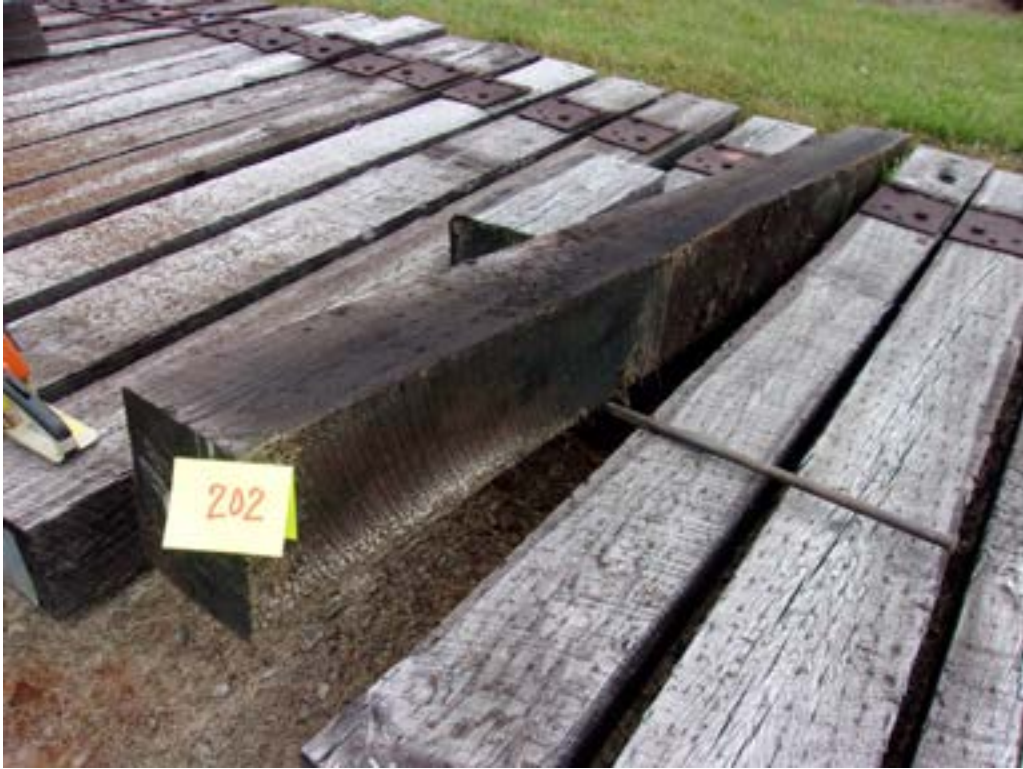
Figure 95 – Tie #202 white oak/borate/creosote 7lbs (Koppers).
