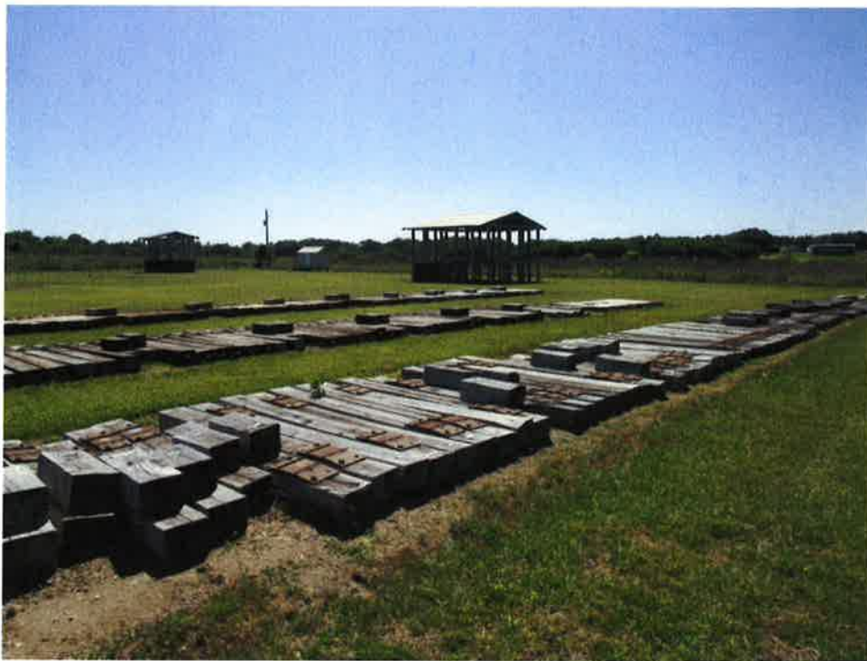
Figure 1 - An overall view of exposure Site 2 illustrating the conditions at the time of inspection.
