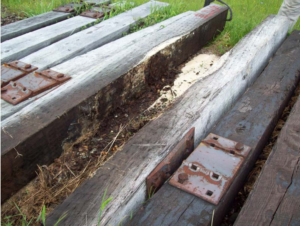
Figure 7 – As shown in this photograph, the harsh conditions of exposure provided ample opportunity for the growth of decay fungi (Site 1).
