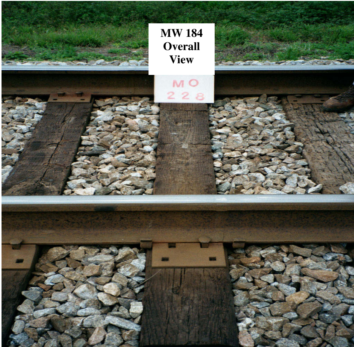
MW 184 Overall View
