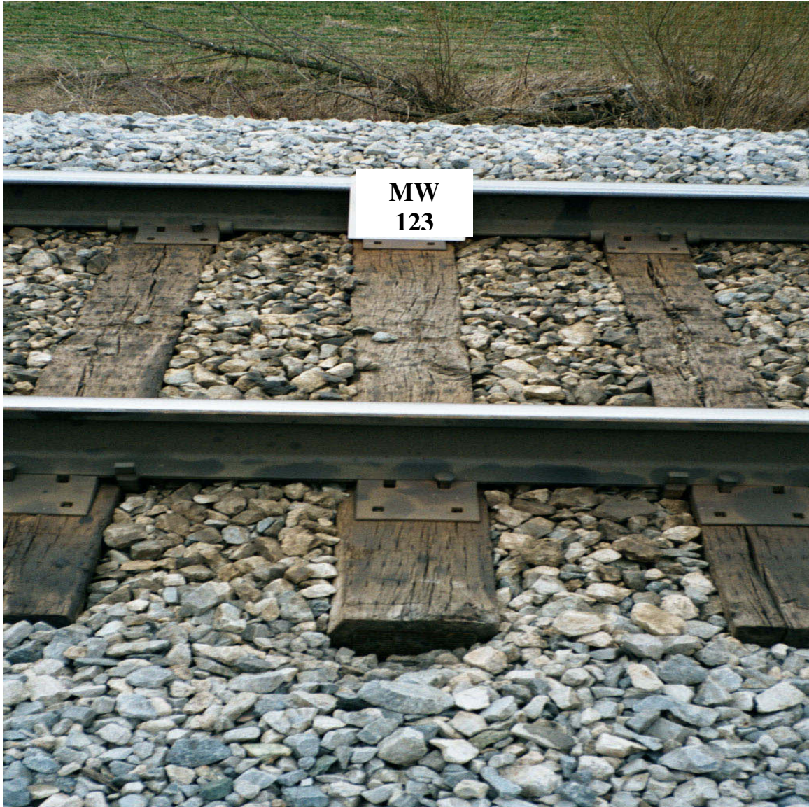
MW 123 Good Tie
