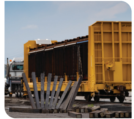
Ties coming off the tie unloading railcar.
