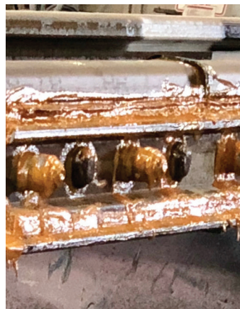
Kevlar and epoxy applied to reinforce.
