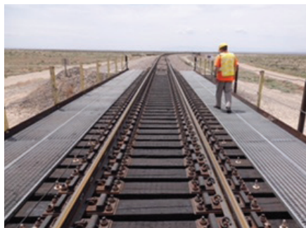
Open-deck bridge ties on the 65-foot span of the East Steel Bridge. The ties are Douglas fir with 10-inch-wide Progress Rail Loadmaster™ plates. Hook bolts are standard J bolts.
