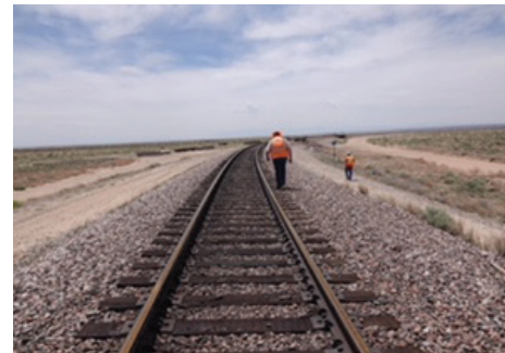
Standard hardwood ties with cut spikes and anchors in open track.
