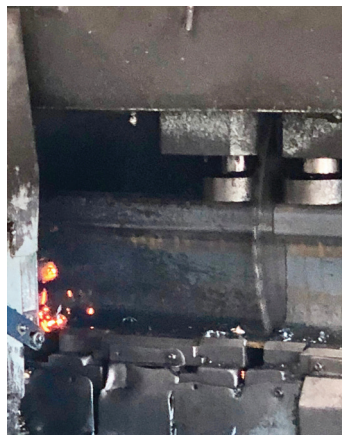
Rail being cut and drilled.
