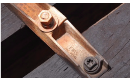
Open-deck bridge ties on the 65-foot span of the East Steel Bridge. The ties are Douglas fir with 10-inch-wide Progress Rail Loadmaster™ plates. Hook bolts are standard J bolts.
