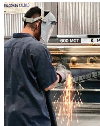
Cleaning the excess prior to painting.
